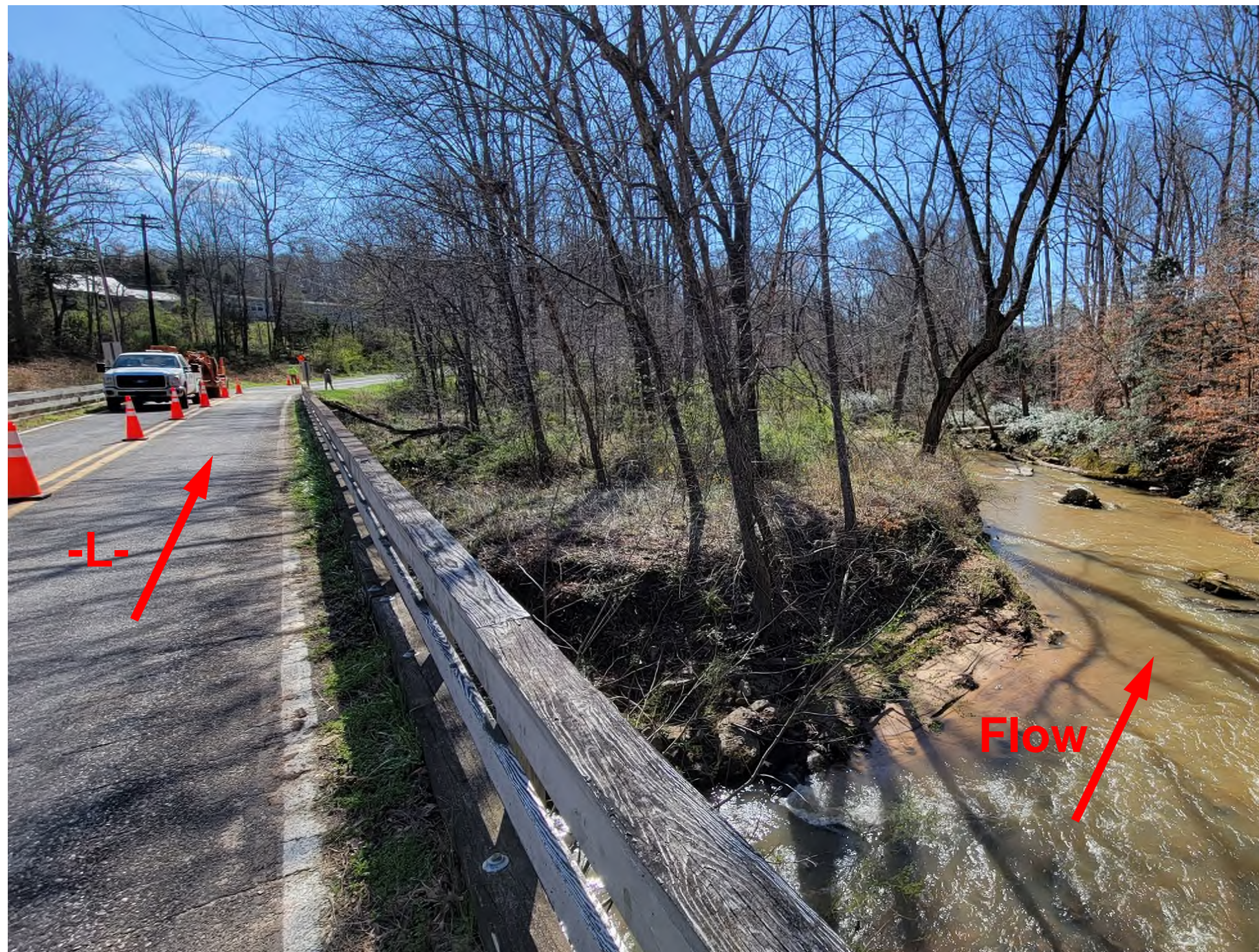
Looking downstation towards Highway 74
